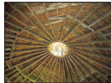
The beautiful skeletal structure of the roof
