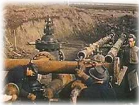
Montreal Pipeline Construction
