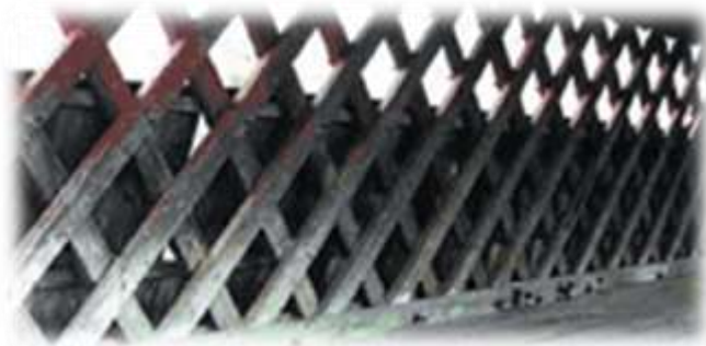
Triangulated beams, simple Town type
