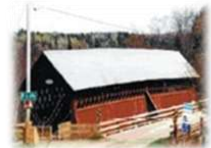
Exterior sheathing protects the structure
